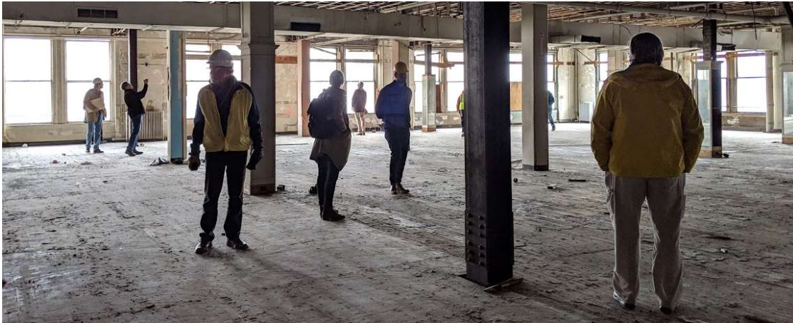
Developers, architects, and engineers evaluate the Brager-Gutman building, 201 W. Lexington Street.
